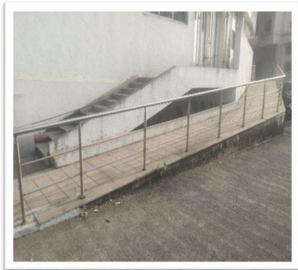
SLOPE/RAMPS FOR WAY TO THE DEPARTMENT
