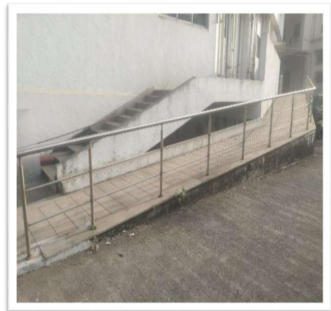
SLOPE/RAMPS FOR WAY TO THE DEPARTMENT
