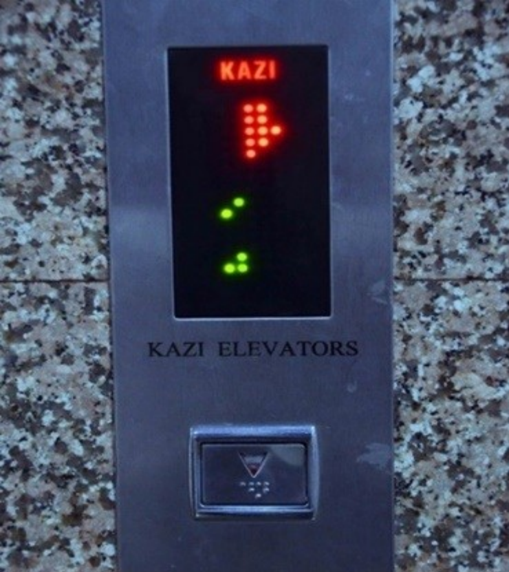
Lift with braille facility, Aurangabad
